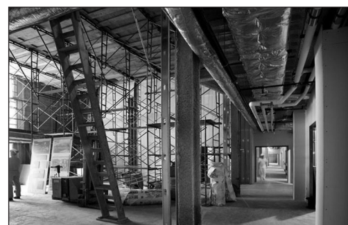
The piping systems were not only constructed but also designed by Heatmasters, a member of the contractor-led design/build team.
